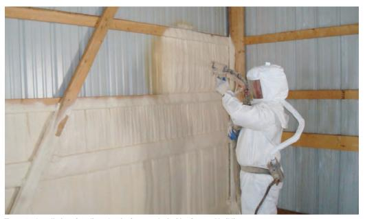
Figure 3-2 Installation of medium-density foam on the inside of a metal building
