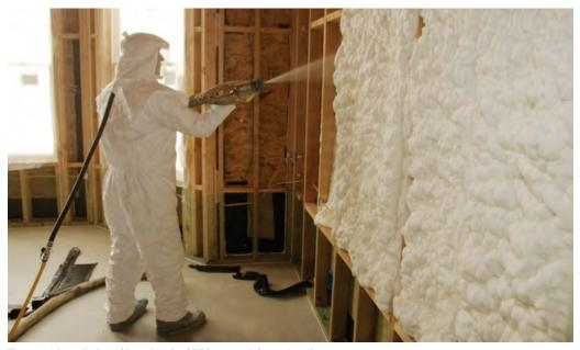
Figure 3-1 Installation of low-density SPF in a wood-framed wall
