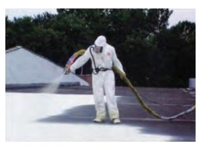
Figure 3-3 Installation of roofing foam on a low-slope roof
